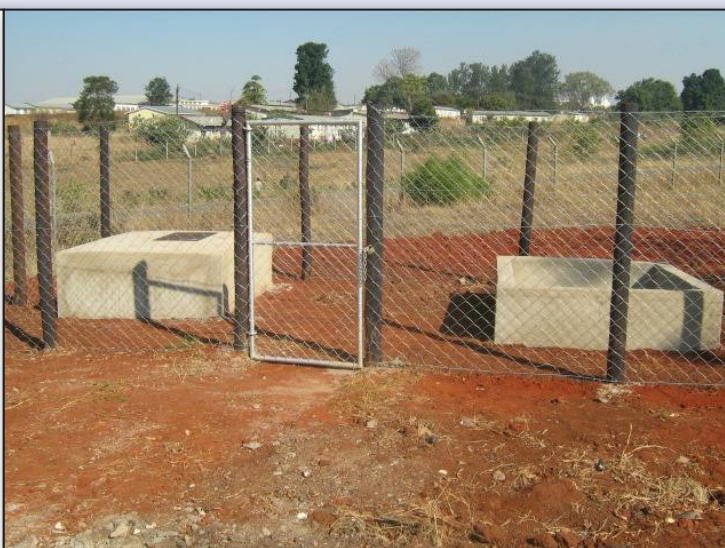
Figure 20: Healthcare waste secured pits.
